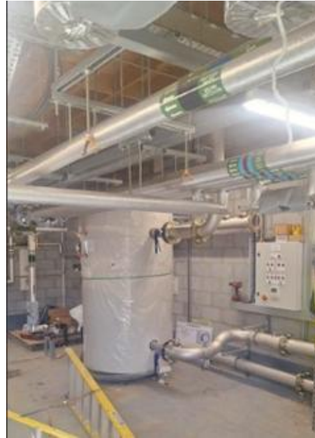
Buffer Vessel, Pumps and control panels inside plantrooms
