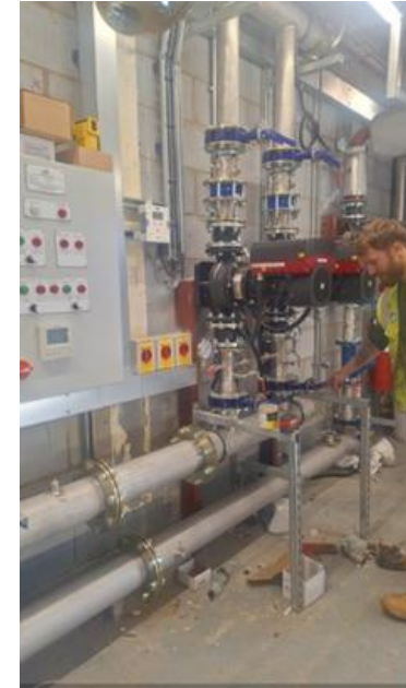
Buffer Vessel, Pumps and control panels inside plantrooms
